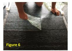
5. Begin laying the LVTs or tiles ensuring the first rows remain in place by checking the alignment is parallel to the centre line of the room. Gently place the LVTs or tiles onto the exposed rubber adhesive membrane. The bond to the adhesive membrane will increase with some downward pressure.
